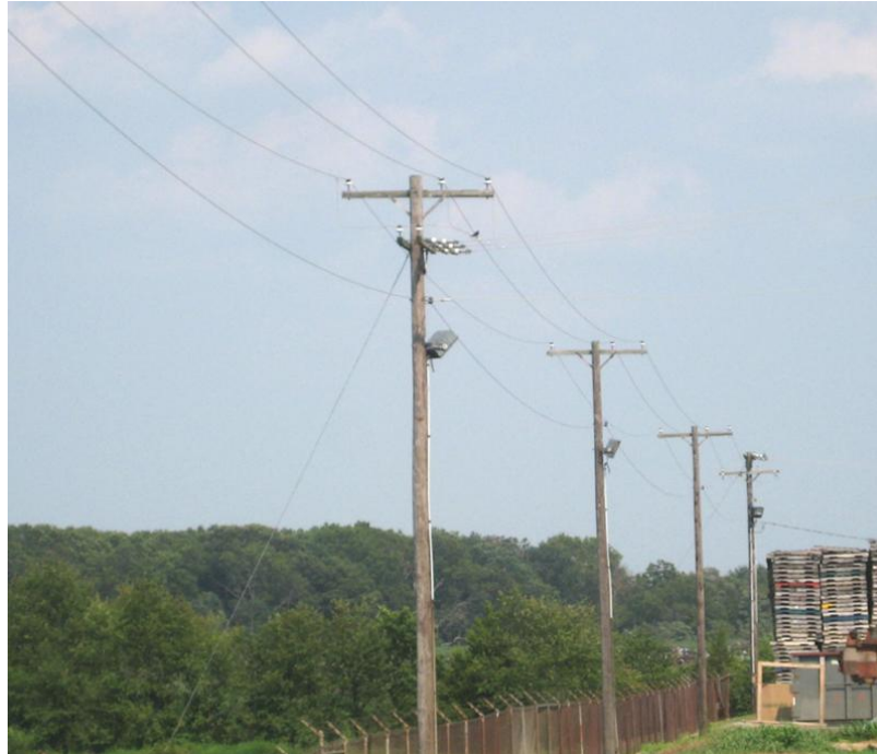
Figure 3. Existing Customer-owned Overhead adjacent proposed site
