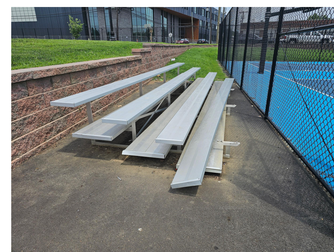
Figure 4. Broken bench at Whitman Park.
