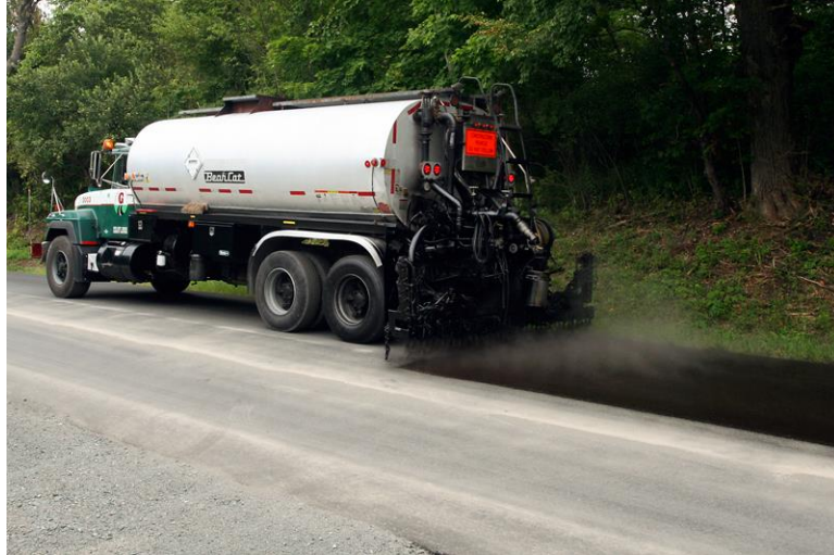
Figure 6. Fog Sealing (The Gourman Group, 2019)
