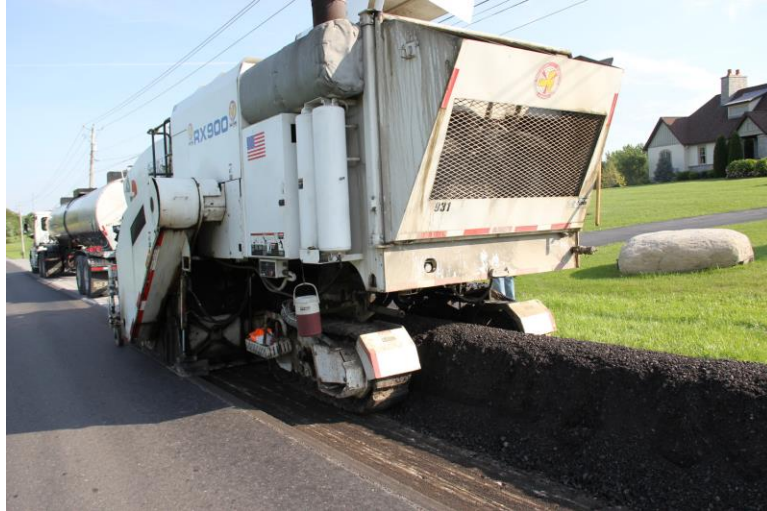
Figure 4. CIR Mix Placement (Suit-Kote, 2019)
