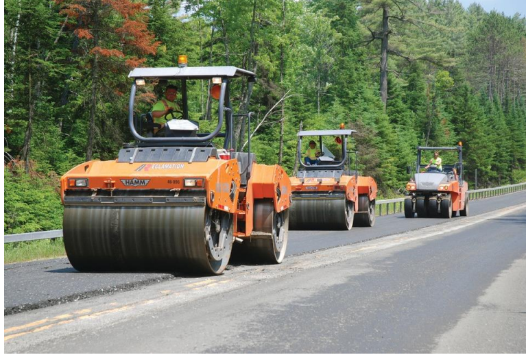
Figure 5. Compaction Process (ForConstructionPros.com, 2019)
