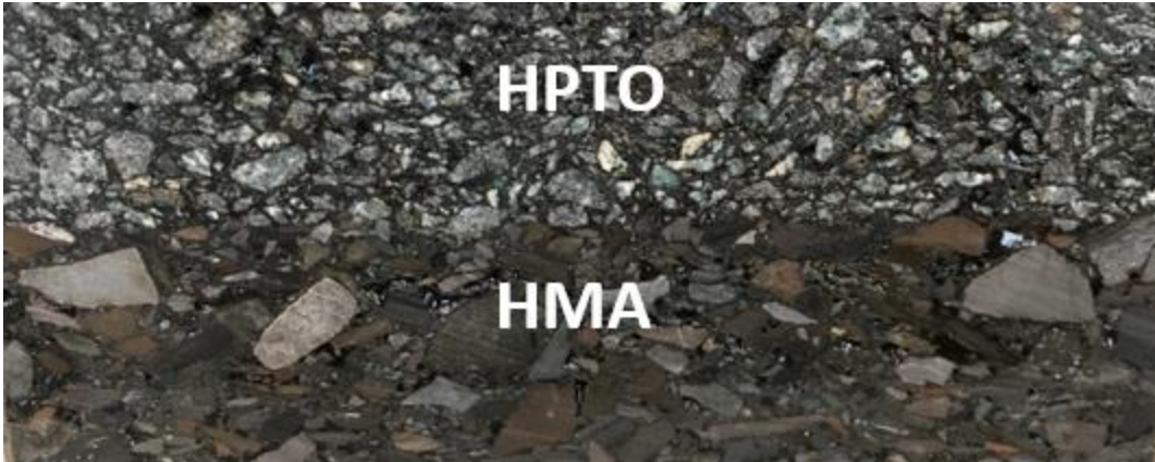
Figure 3. Thin-overlay applied to HMA.
