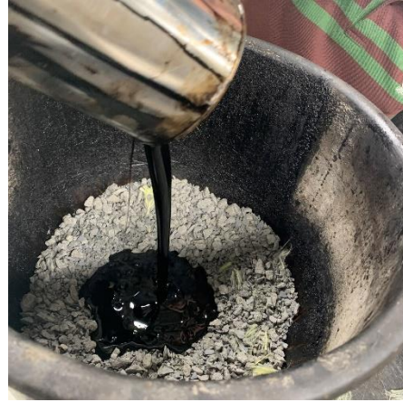
(b) Addition of asphalt binder
