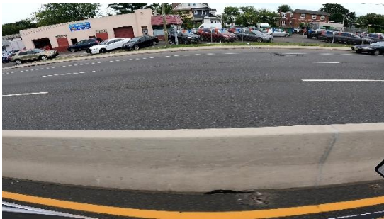
c) Positive Median (concrete)
